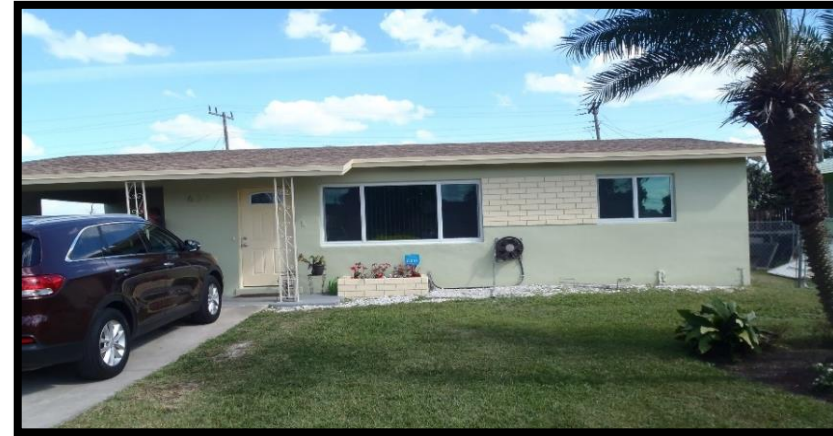
Single-Family Rehabilitation, Belle Glade
